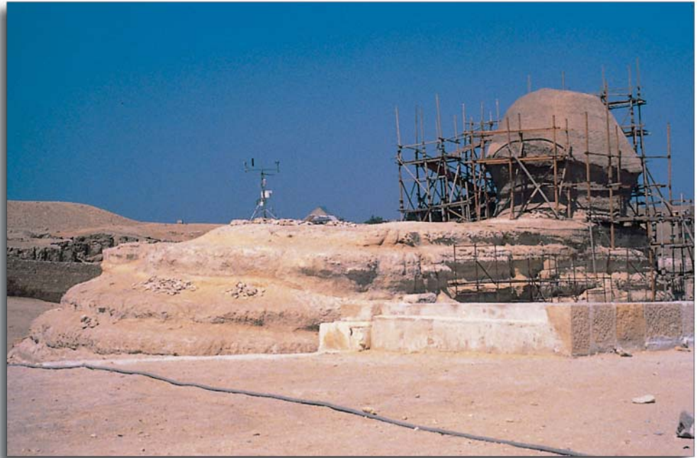
A weather station provides environmental data needed for the restoration and preservation of the Sphinx. Continuous monitoring of meteorological parameters provides crucial information for managing and preserving outdoor sites.
