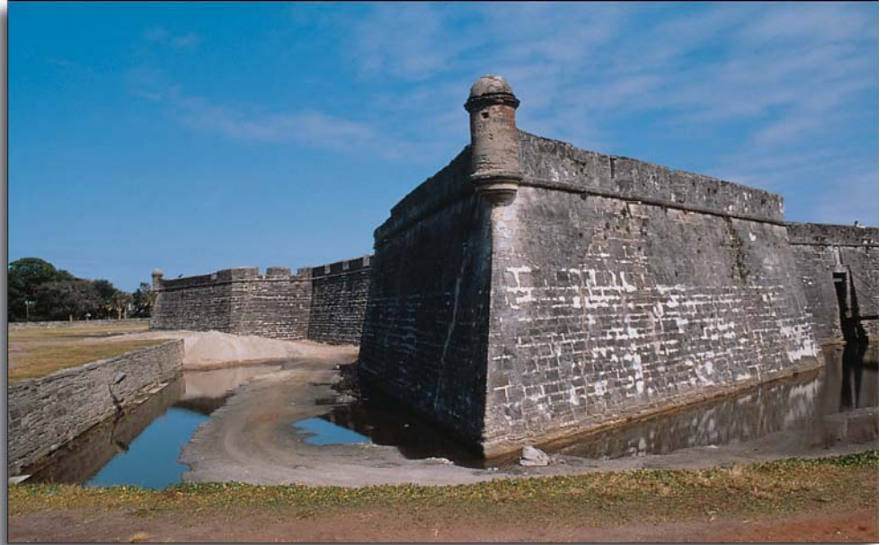
A preservation project at Castillo de San Marcos, St. Augustine, FL involves monitoring cracks in three dimensions, the tilt of the large segments between the major cracks, change of soil moisture within the bastion, and weather conditions at the site.
