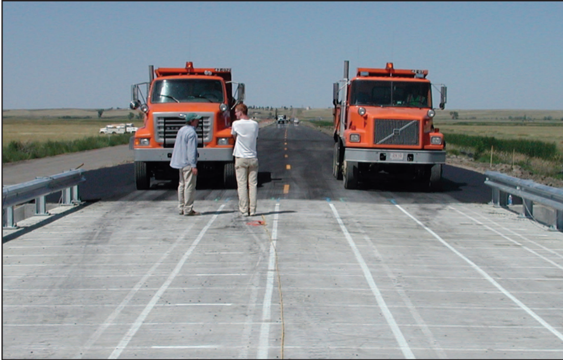
Researchers prepare for a two-truck live load test in order to reach one of the objectives of the Montana highway project, which is to compare load-carrying mechanisms of three different bridge decks near Saco.
