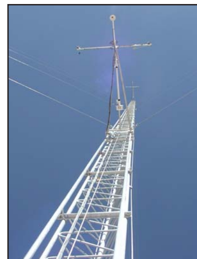
View of two deployed instrument platforms from below; the wind speed, wind direction, and aspirated temperature sensors can be distinguished.
