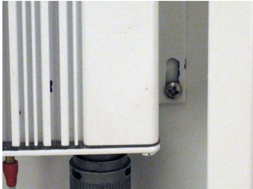
FIGURE 2. Proper mounting position of the electronics box.
