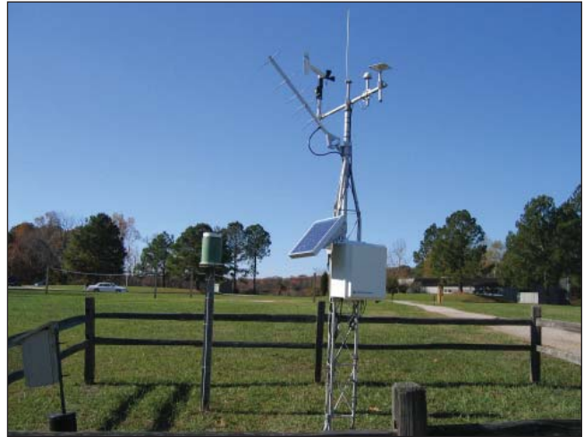
This station for the National Estuarine Research Reserve (NERR) in Virginia transmits data via our GOES satellite transmitter.
