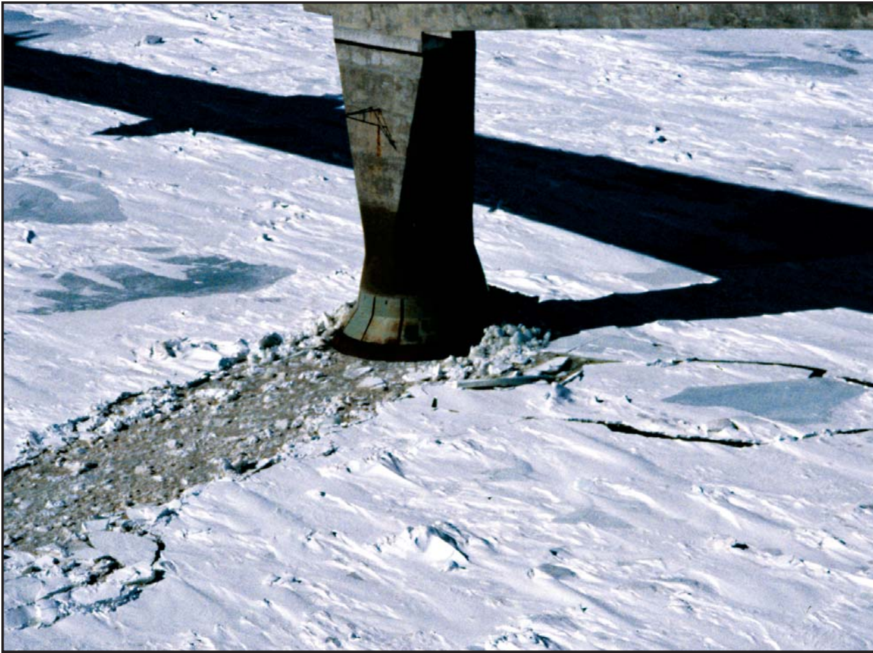
The force of ice floes impacting the bridge and the bridge's response to the impacts are monitored by two CR9000 systems.
