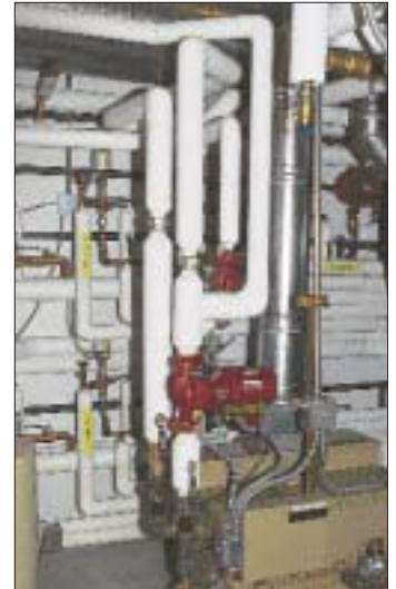
Systems can monitor and control pumps, fans, and starter motors. Proportional control of dampers is also possible.
