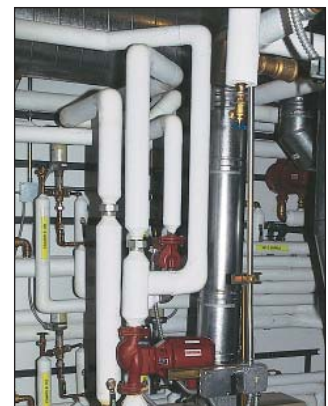
The CR3000 can monitor and control pumps, fans, and starter motors in an HVAC system.
