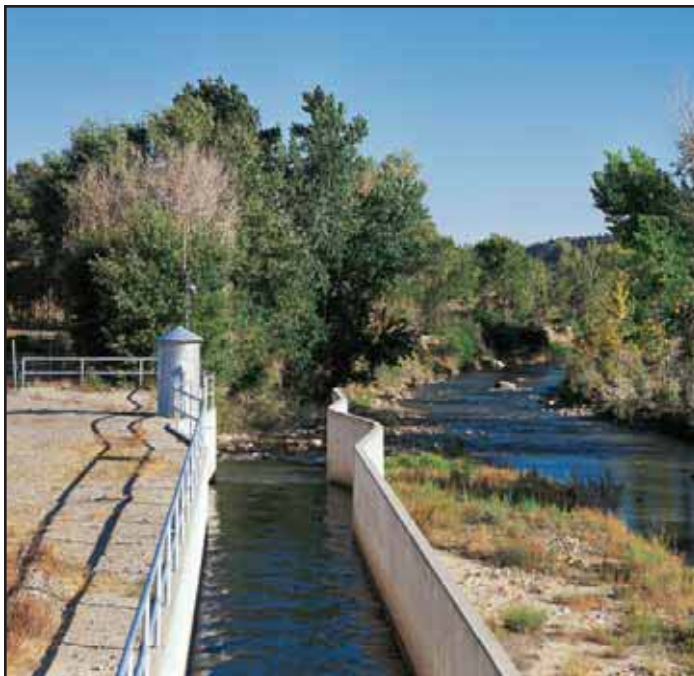
Datalogger measures water level using a shaft encoder, then calculates flow. The data are telemetered, via radio, to the water master for further processing, review, and archive. Stilling well at diversionary dam, Emery County, Utah.
