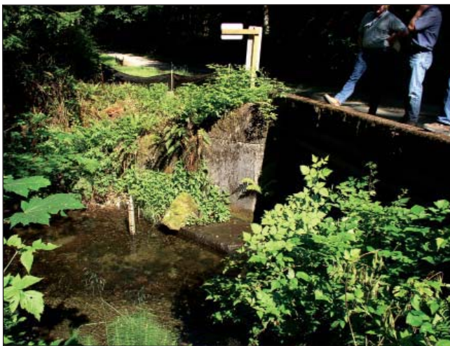
A turbidity sensor was installed in a tributary of the Cedar River watershed to monitor water quality conditions for the city of Seattle, Washington.
