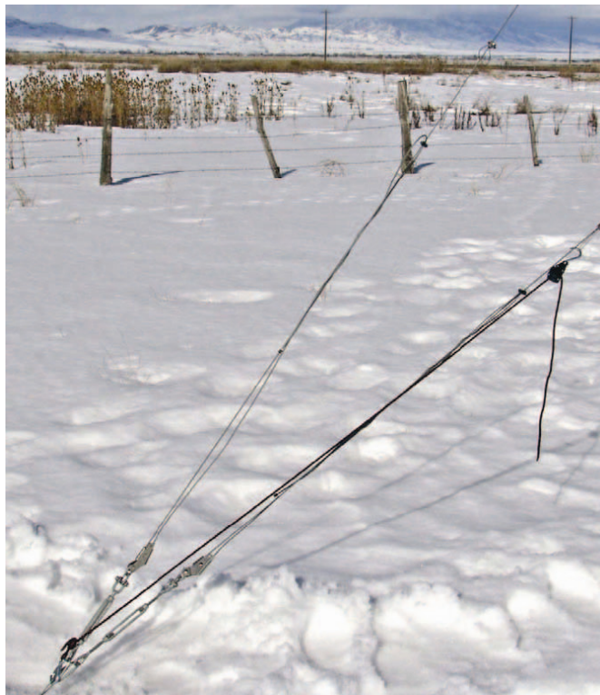
FIGURE 2.4-8. Rope Ratchet Assists Assembly
