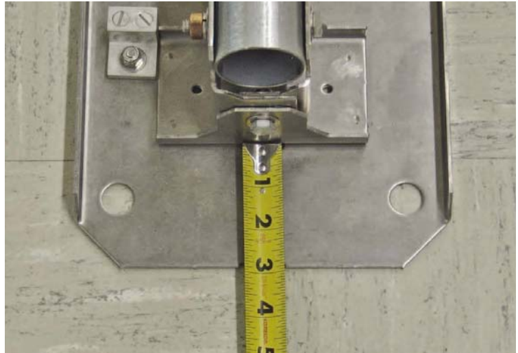
FIGURE 2.4-1. Tape Measure in Slot for South Anchor
